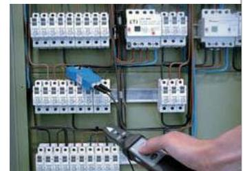
This tracing method uses A1074 current clamps. The high accuracy of this method allows for pinpoint determination of a wire or fuse without removal of the plastic cover of the switch box.
