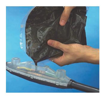
**3M<sup>™</sup> Scotchcast<sup>™</sup> Resin Joints** offer a high degree of mechanical strength for physical protection of connections and moisture-resistant insulation in above ground or direct burial applications.
