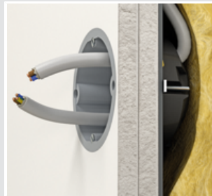
The one-gang junction box is now ready for use.
