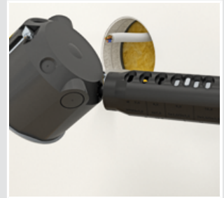
Use the universal opening cutter (Art. No. 1085-80) to cut the matching conical opening.
