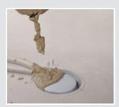
... fill the free space with concrete and compact it. A formwork board fitted underneath prevents the concrete from running out.
