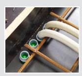
The small design also allows many exits on a small wall or ceiling area.
