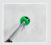
After striking the formwork, use a screwdriver for fast, easy opening of the plaster skin.
