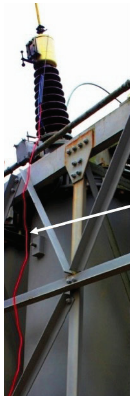
Screened cable running down the side of a transformer to the insulation tester.
