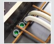
The small design also allows many exits on a small wall or ceiling area.
